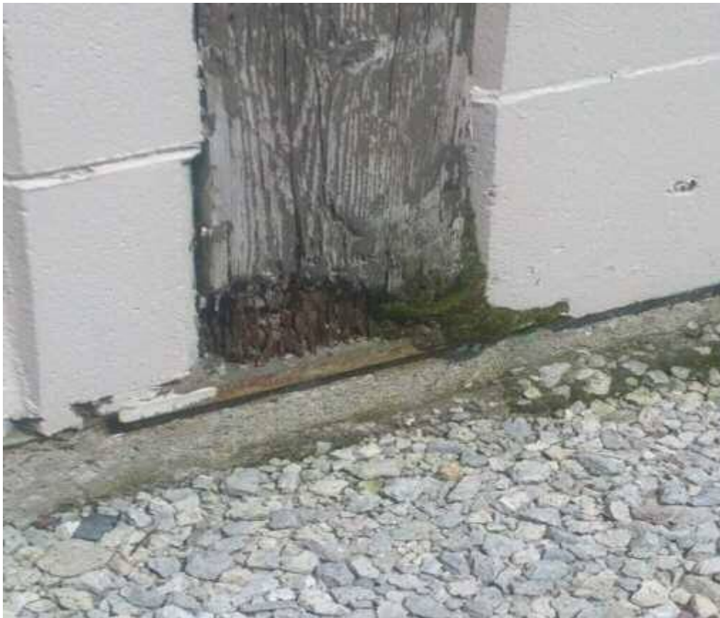
Photo 13 – Exposed Timber Columns (South Side)
