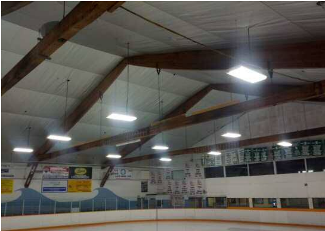
Photo 11 – Existing Timber Roof Trusses (Ice Surface)
