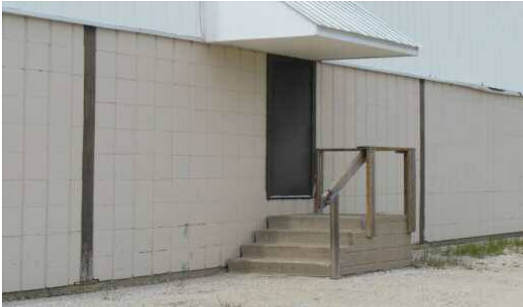
Photo 8 – Exterior Exit Door (South Side of Arena)
