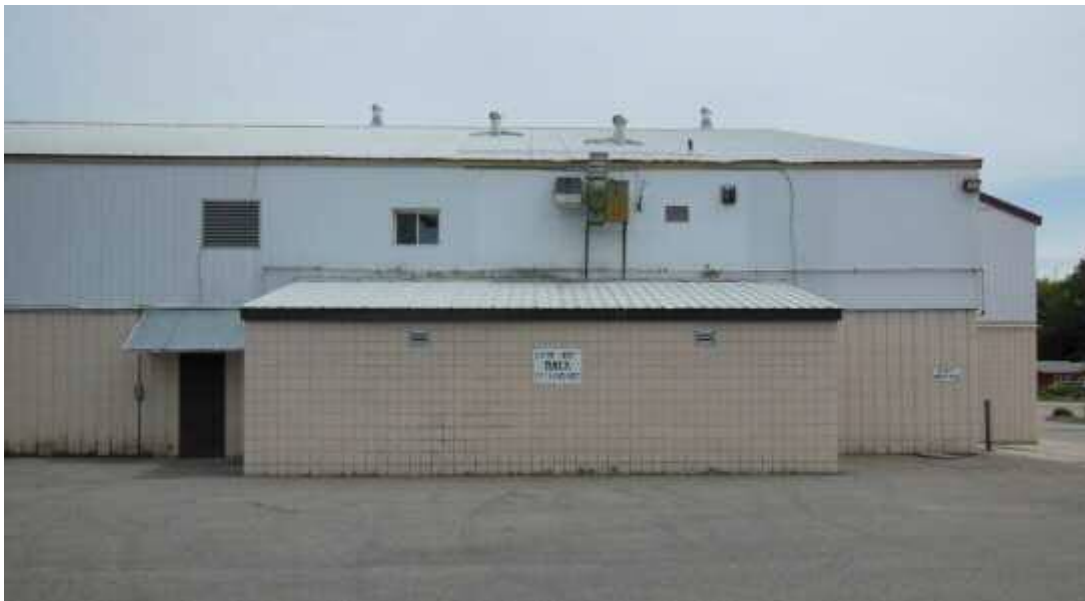
Photo 7 – Standing Seam Metal Roofing (Dressing Room Nos. 1 & 2)
