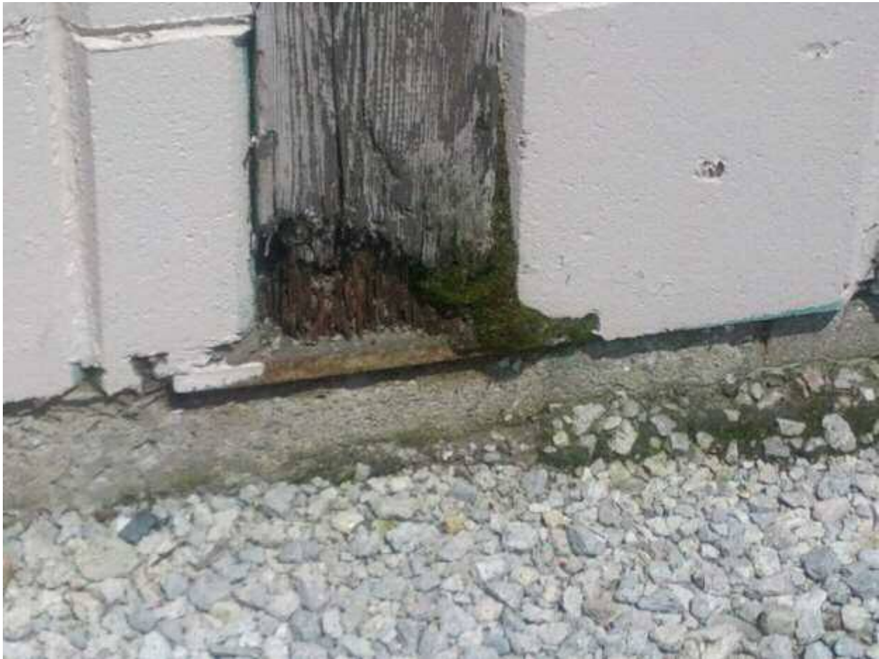
Photo 14 – Exposed Timber Columns (South Side)
