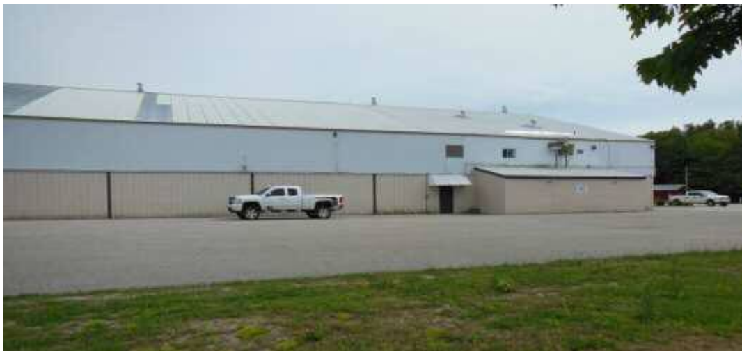
Photo 6 – Standing Seam Metal Roofing (North Side of Arena)
