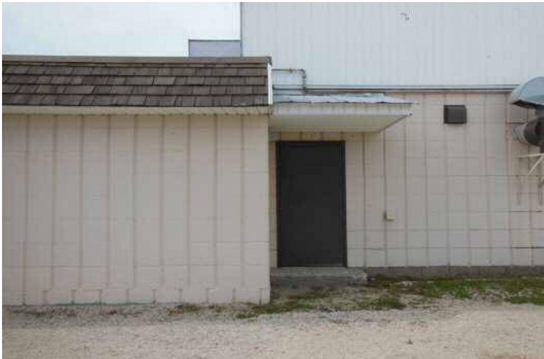
Photo 3 – Existing Exit Door at South Side of Building
