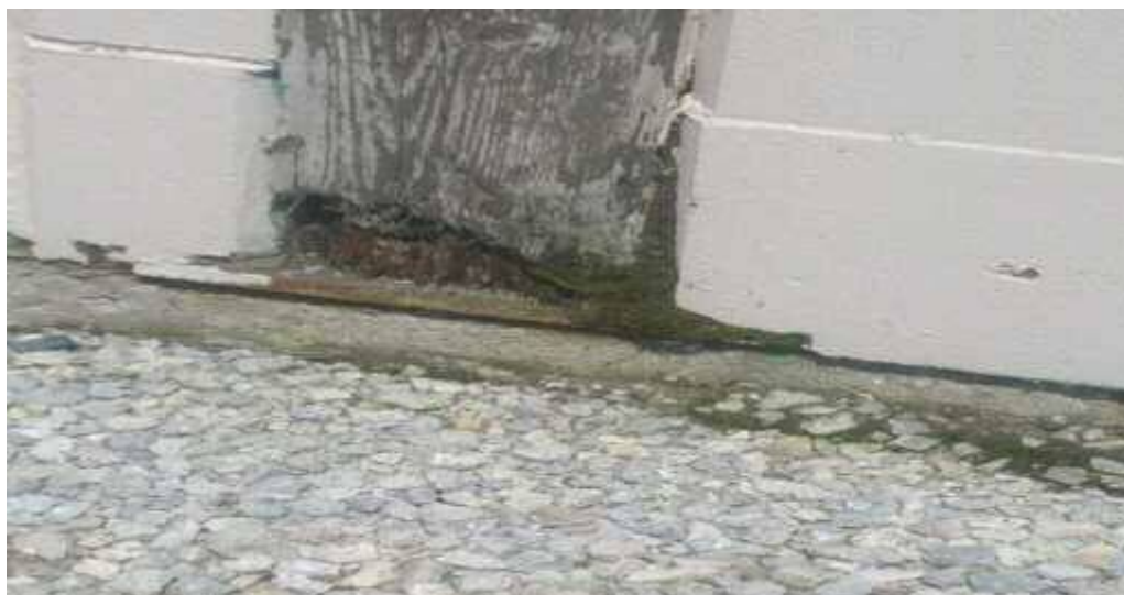
Photo 10 – Exposed Timber Columns ( North & South Sides)
