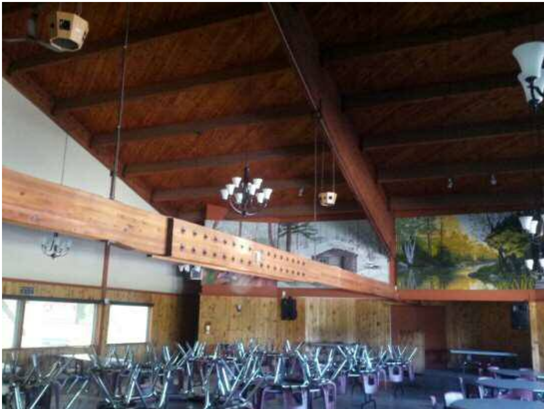
Photo 12 - Existing Timber Roof Trusses (Upper Level Hall / Auditorium)
