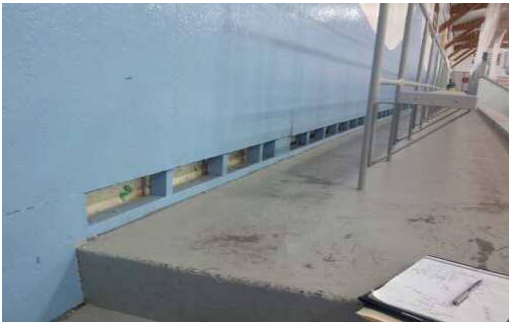
Photo 5 – Spectator Seating / Standing Area (North Side)
