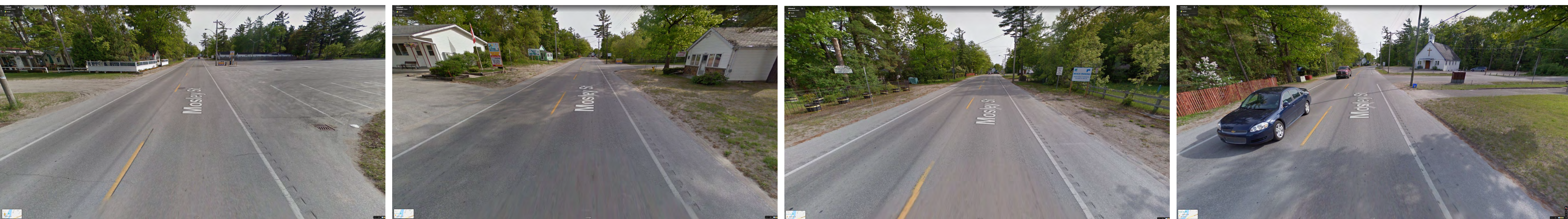
MOSLEY STREET - 3 rd Street to 6 th Street
