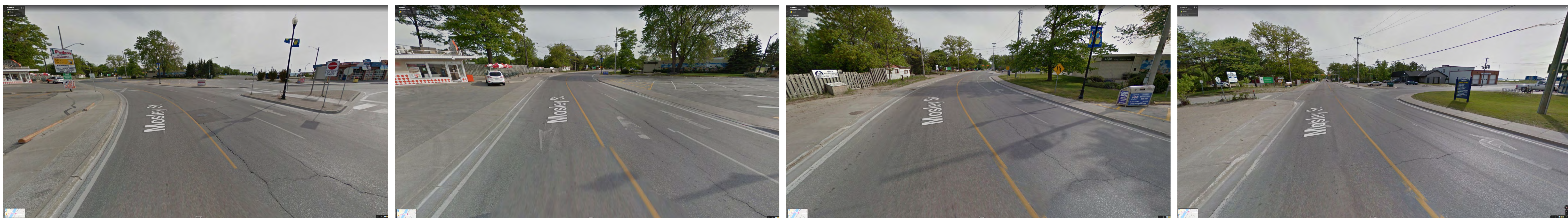
MOSLEY STREET - 1 st Street to 2 nd Street
