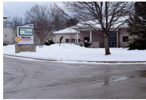
Wasaga Distribution is the local utility provider in Wasaga Beach. It provides electricity needs throughout the community.
